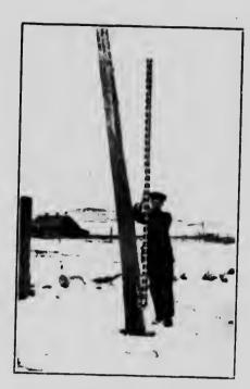
Photo by J. N. Wallawe, D.L.S. T.B.M. on spike on telegraph pole,
