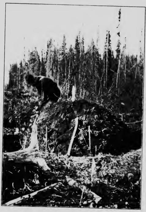
Photo by J. A. Fletcher, D.L.S. Witness mound. Established when the corner of a section falls in a lake or other inaccessible place, 73075—p. 128.
