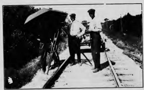
$\label{eq:photo-by-L} Photo-by-L,\,O,\,R,\,Dozies,\,D.L.S.$  An instrument station, Precise Levelling.
