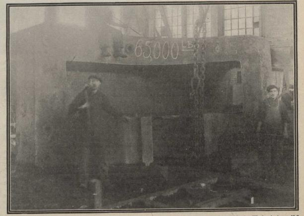
321/2 Tons of Iron in a Single Casting for a Rolling-mill Engine; Produced at the International Engineering Works, Amherst, N.S.
