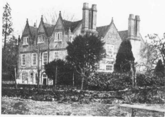
QUEBEC HOUSE, WESTERRHAM
