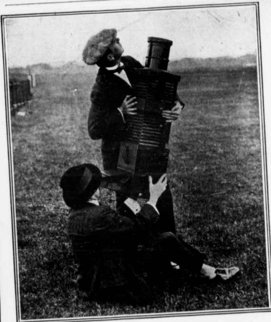
HOW A HIGH-FLYING AEROPLANE IS PHOTOGRAPHED: "LONG TOM"— A TELESCOPIC CAMERA.
