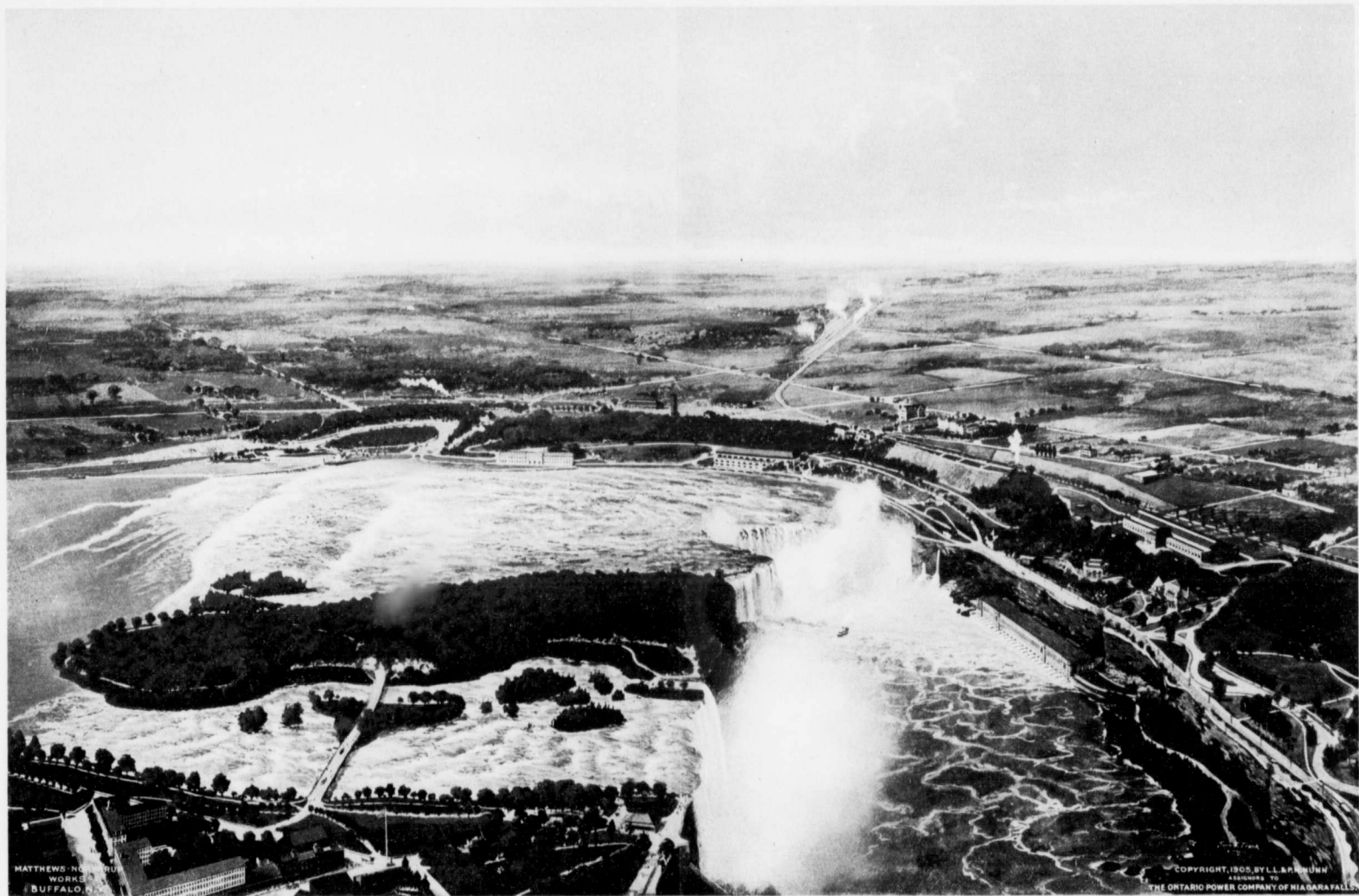
BIRD'S EYE VIEW OF NIAGARA FALLS SHOWING POWER DEVELOPMENTS ON CANADIAN SIDE.
