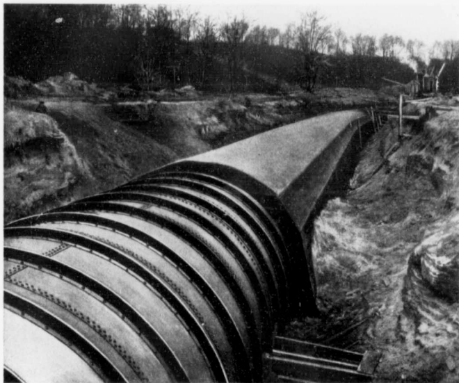
EIGHTEEN FOOT DIAMETER CONDUIT SHOWING CONCRETE ENVELOPE.
