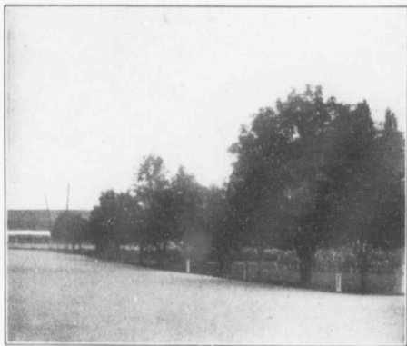
Entrance to Church Park.
