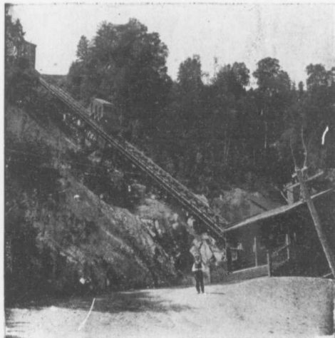
Passenger Elevator, Montmorency Falls.
