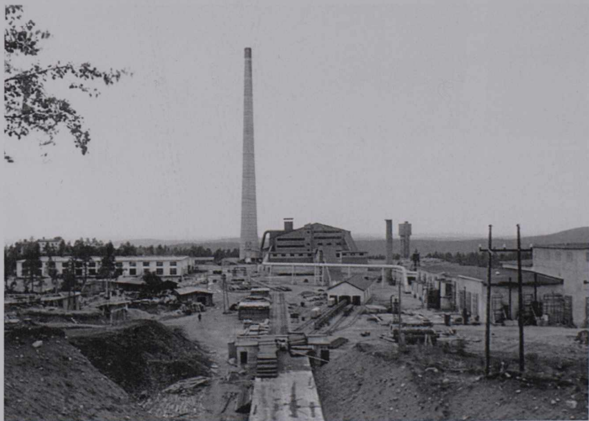
Kolosjoki nickel and copper mine area and buildings, Petsamo. Smelter with 165-metre smokestack (highest in Europe at the time). Photo: Kalervo Rankama, 1942. Source: Open licence of the Geological Survey of Finland. Old photos #5810.
