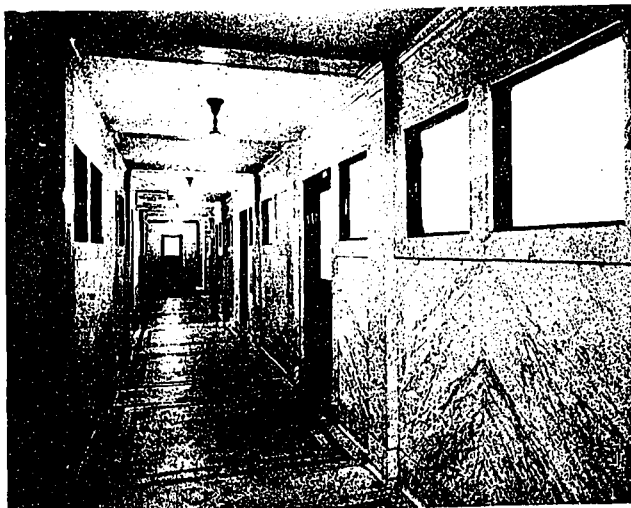
TYPICAL CORRIDOR, EXCELSIOR LIFE BUILDING.
