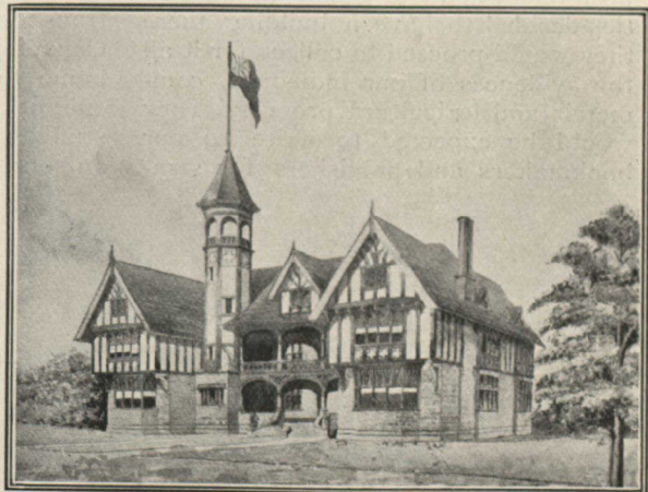
CANADIAN BUILDING AT THE PAN
