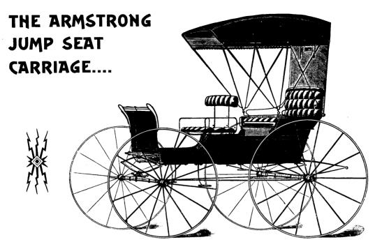
Arranges instantly as a One-Seated Buggy or with Seat against Dash. Easy back turning. The best Gear for this purpose is the Armstrong "Monitor" under this Carriage.
