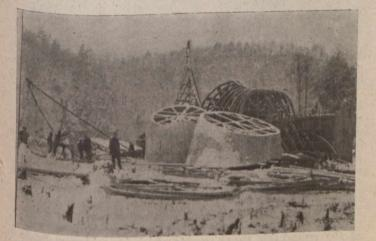
DRAFT TUBE FORM CUT IN SECTIONS TO FACILITATE MOVING, APPALACHIAN POWER CO.
