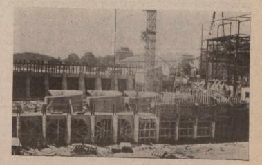
SCROLL CASE AND DRAFT TUBE FORMS IN POWERHOUSE AT MINETTO, N.Y.
