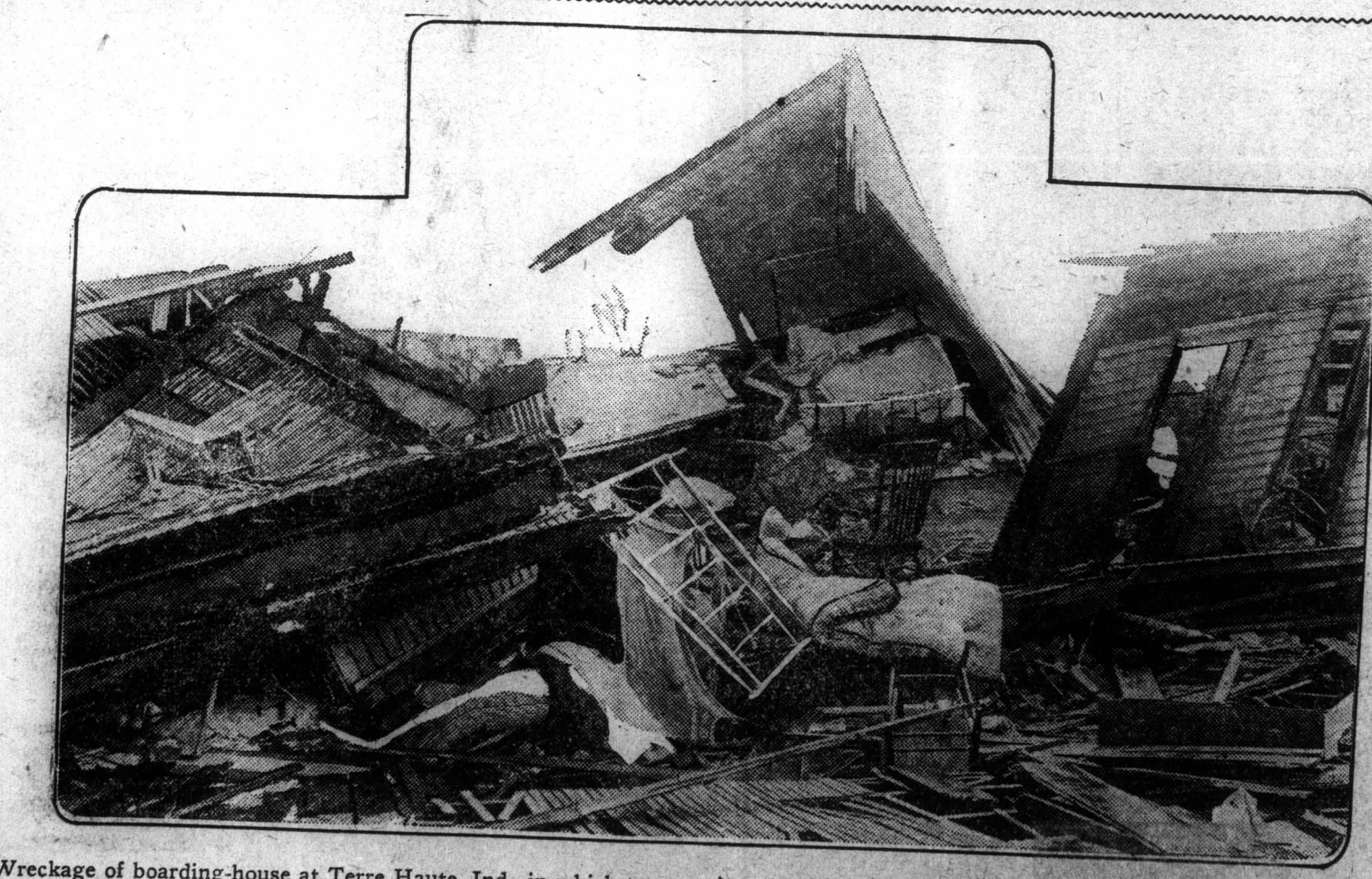
Wreckage of boarding-house at Terre Haute, Ind., in which ten people were caught. Two were killed. About 250 houses were wrecked.
