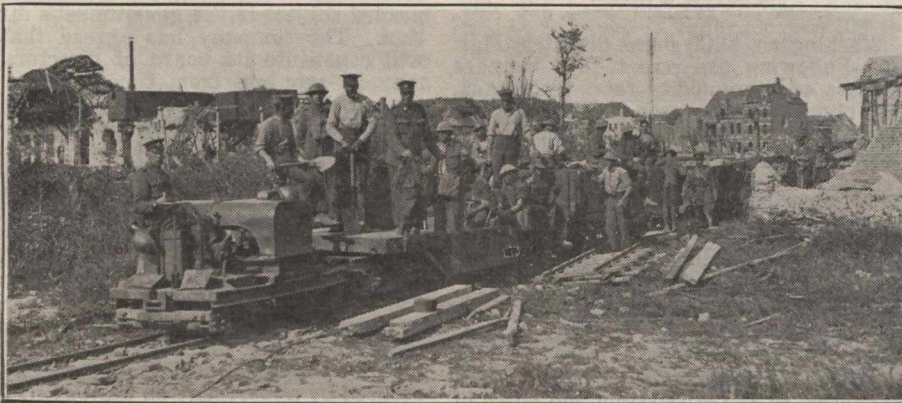
On the Western Battle Front. Canadian Railway Troops passing through the ruins of a town after laying track. From Canadian official photograph loaned by C.P.R.
