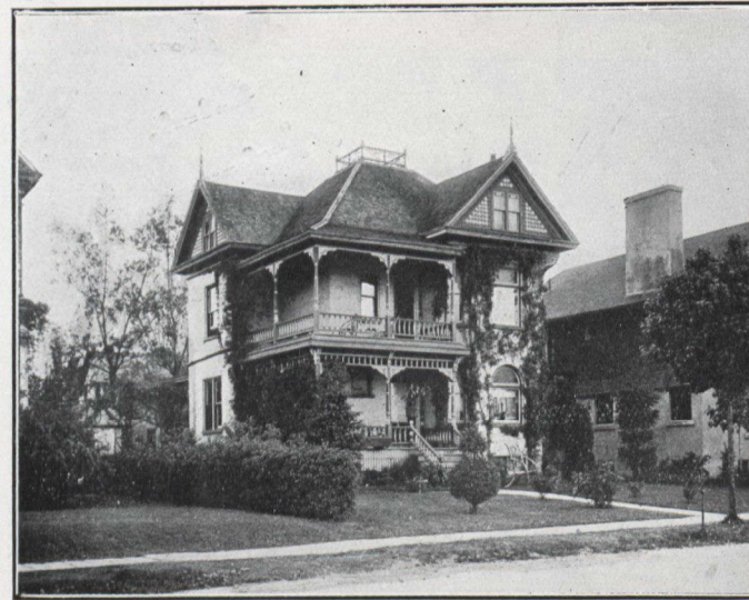
Residence of John Derbecker, 33 Roland St.
