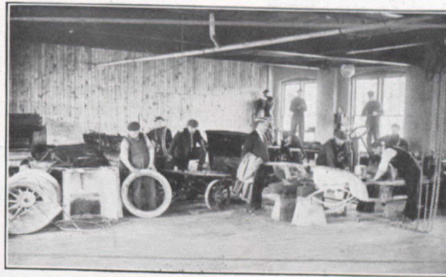
REPAINTING AND REPAIR FLOOR
