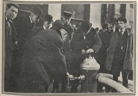
Watching the cyclometer. The indicated pressure before the test was 300 lbs.; when six streams were turned on it fell to 225.
