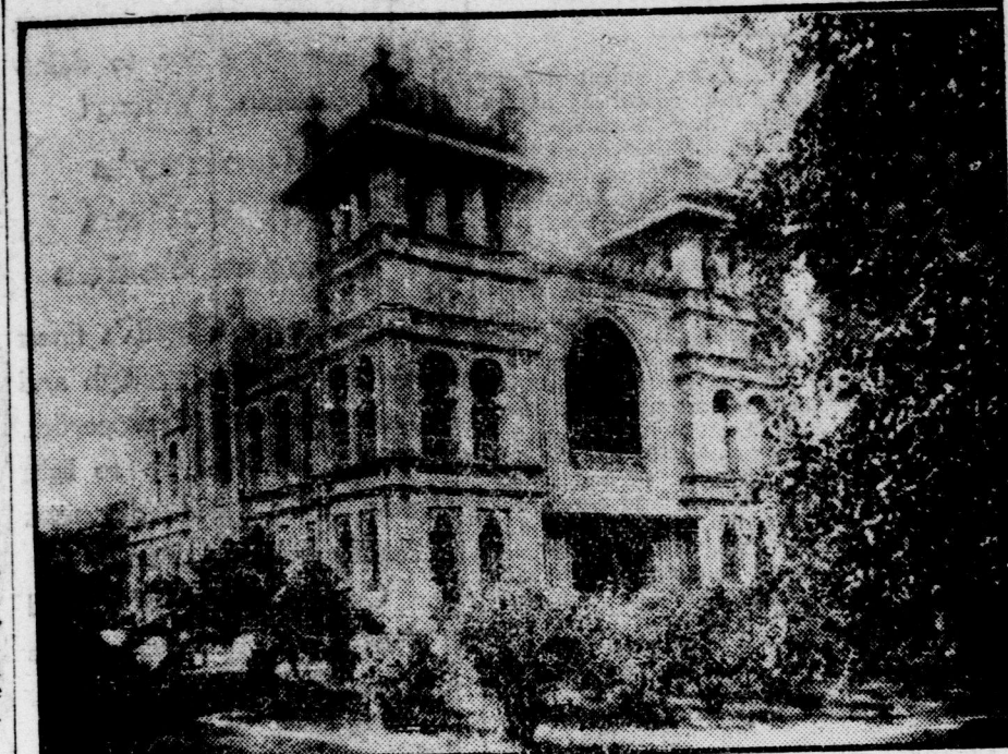
THE TOWN HALL AT LAHORE, INDIA, RUINED BY THE RECENT EARTHQUAKE.
