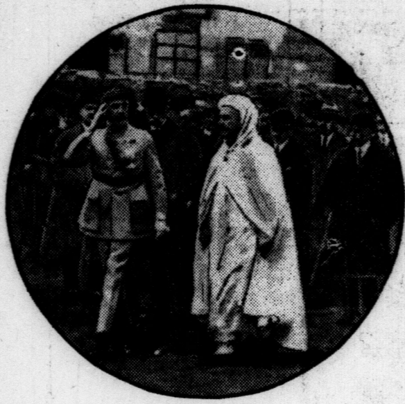
A Moslem mosque is being built in Paris. Marshall Liautey is shown here arriving with the Mohammedan representative, Si Kaddour Ben Chabrit, for the laying of the cornerstone.
