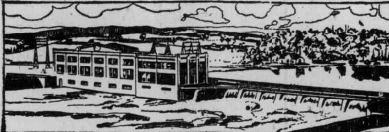
No. 1 Power House, Peterboro, Ont.
