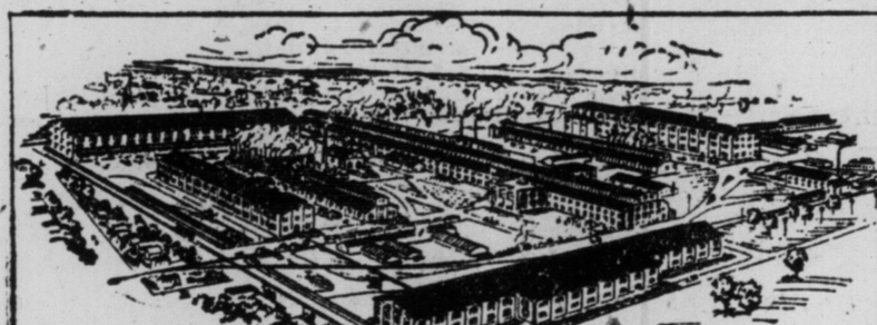
Main Electrical Works, Peterboro, Ont.
