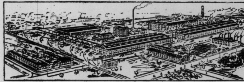
Davenport Works, Toronto, Ont.
