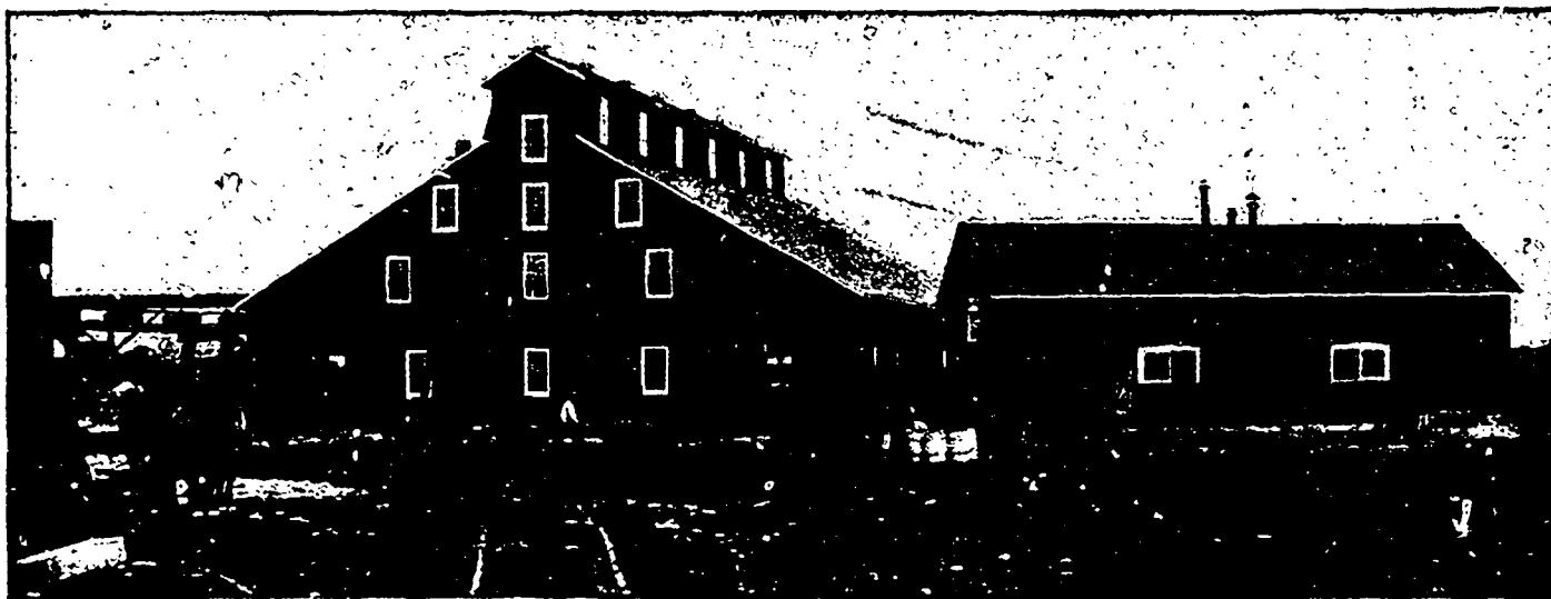
PLANING MILL AND BOX FACTORY OF J. W. HOWRY & SONS, FENELON FALLS, ONT.
