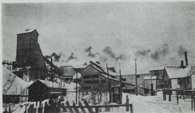
No. 1—General View of Coniagas Mine.
