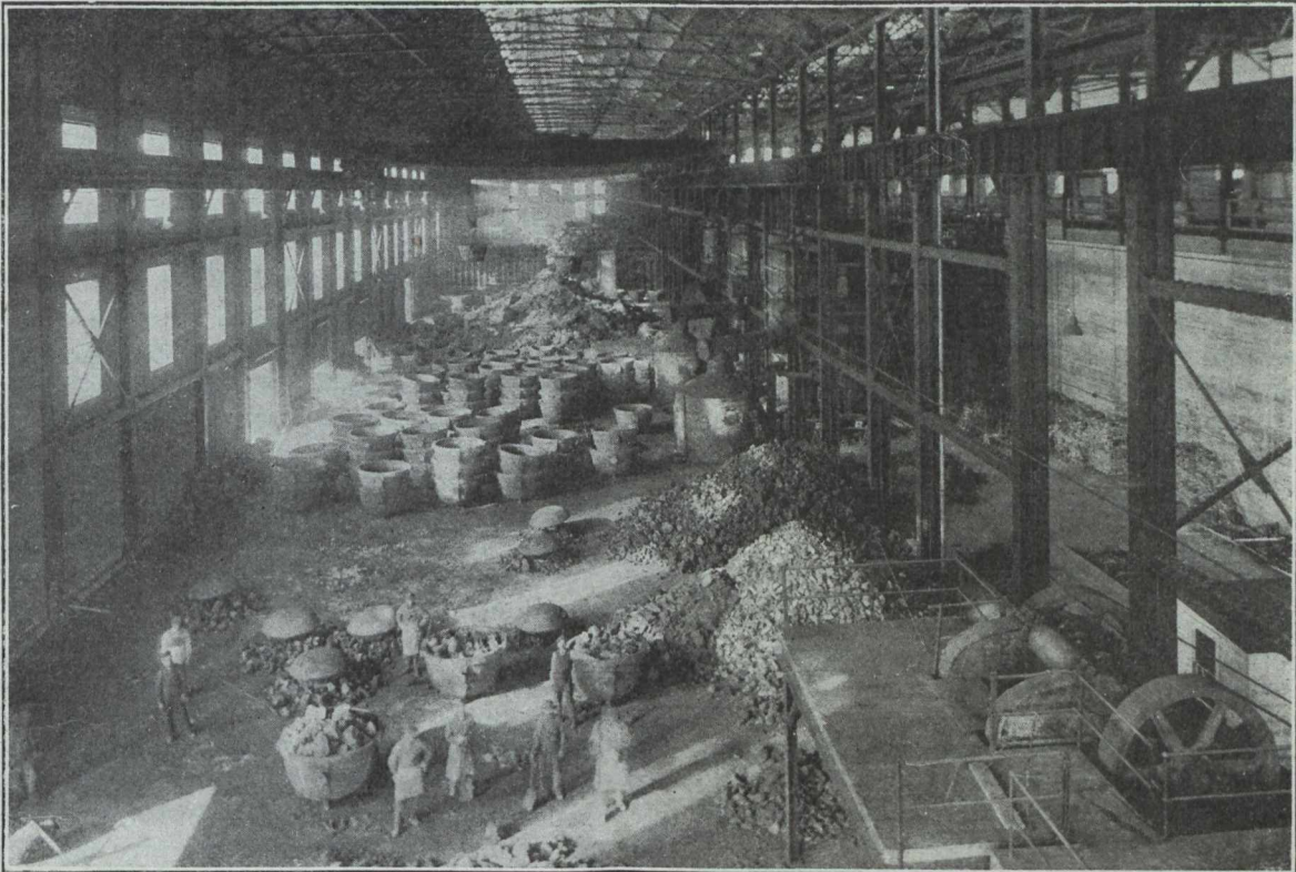
Cupola Building in the Port Colborne Refinery of the International Nickel Co.
