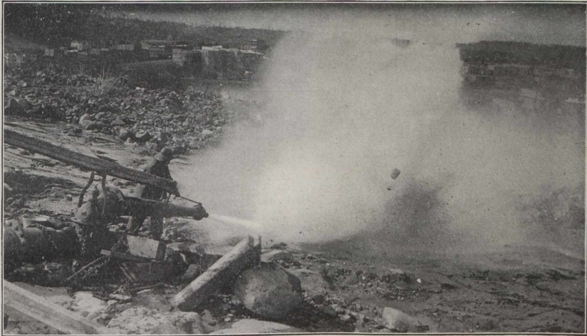
Cleaning Rock Surface, Nipissing Mine
