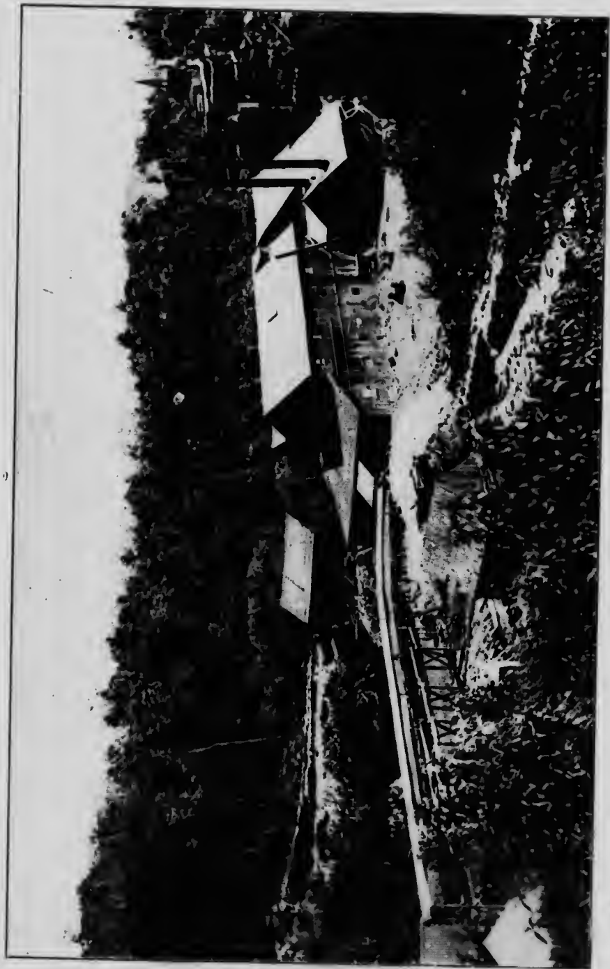
Mill of the Buckingham Graphite Company (North American mine), township of Buckingham, Que. The photograph was taken some years ago, and the buildings are now in a dilapidated condition. The strike of the ore-body is indicated by the tramway, and the main drift enters the mill to the left of the kiln.
