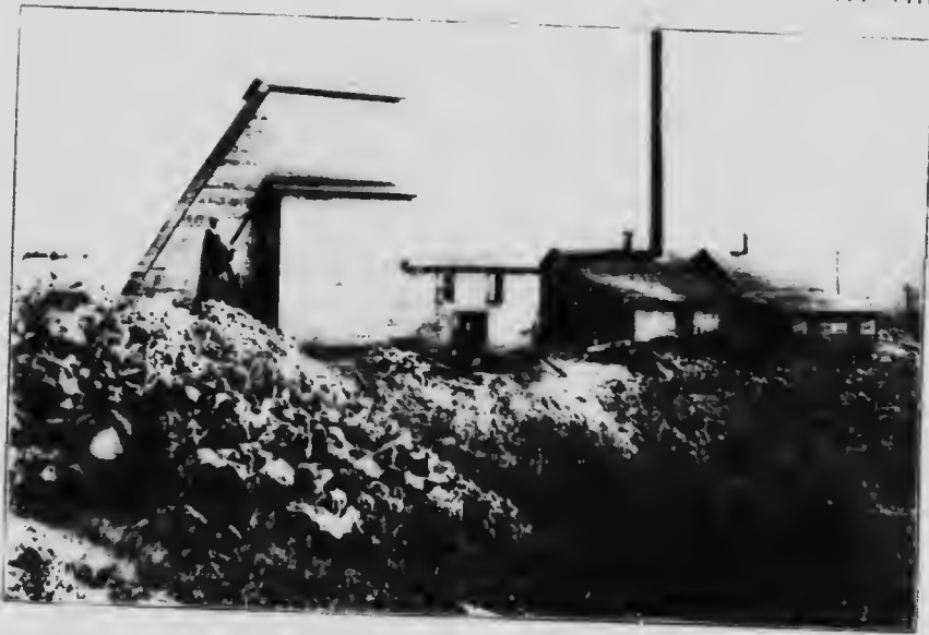
Surface Shaft and Equipment of Pit No. 1 of the Black Lake Chrome and Asbestos Co., Que.
