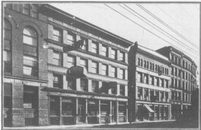
SOME OF THE EIGHTY BUILDINGS DESTROYED—FRONT ST., NORTH SIDE
