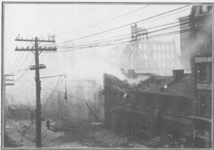
THE FIRE SWEEPED UP BAY ST. TO SOME LOW BUILDINGS NEXT TO THE TORONTO ENGRAVING CO. THESE LOW BUILDINGS ENABLED THE FIREMEN TO STOP THE NORTHWARD PROGRESS AT THIS POINT
