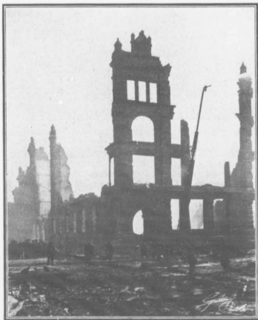
CORNER OF BAY AND WELLINGTON STS.—WATER TOWER AT WORK
