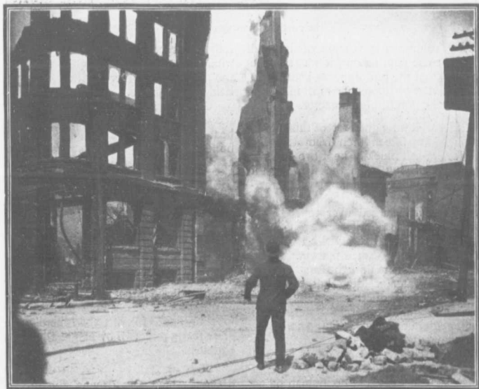
Dynamiting the dangerous walls after the fire—Photo taken at instant of the explosion.
