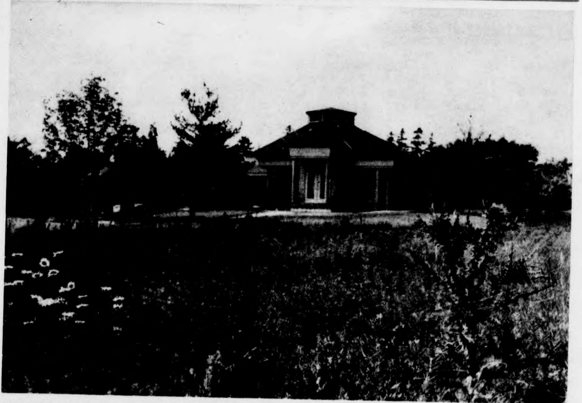
A field of weeds and a decaying sales pavilion, located to the south of the York graduate residences, are all that exist of Bramalea Corporation's ambitious Fountainhead project. The company's glossy brochures showed high-
