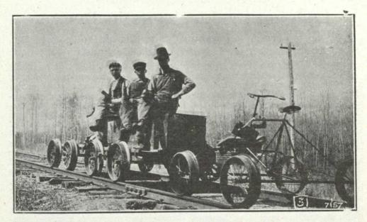
A "track automobile" of the Dominion Forestry Branch in Alberta, showing the motordriven speeder and the velocipede.
