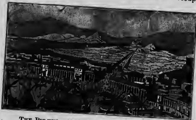
THE PIRÆUS, THE PORT OF ATHENS (Restoration)
