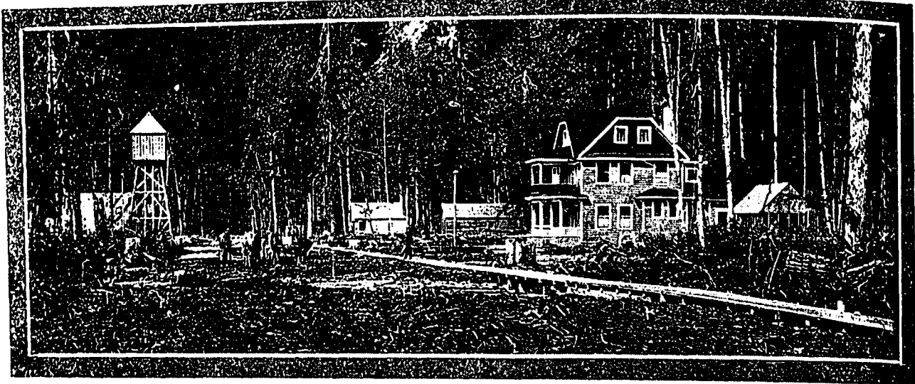
Stewart General Hospital and Water and Electric Light Plant
