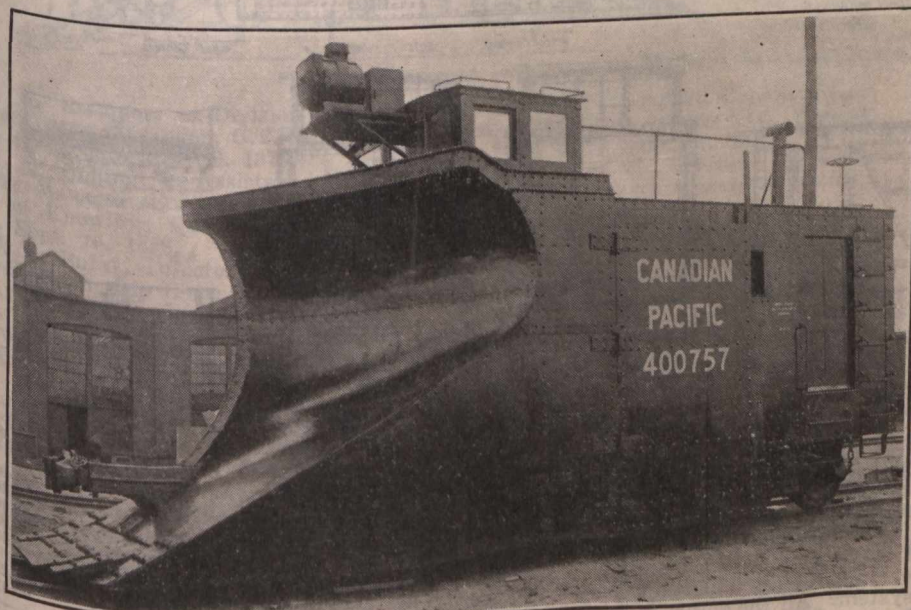
Fig. 13. Single track, steel snow plough, Canadian Pacific Railway. See page 471.
