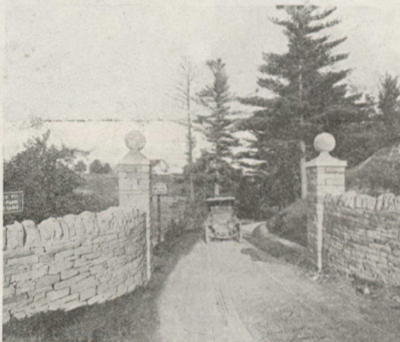
One of the Entrances to Lawrence Park, a Model Suburb in North Toronto.
