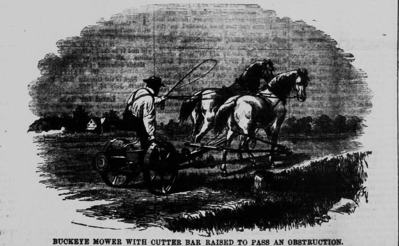
BUCKEYE MOWER WITH CUTTER BAR RAISED TO PASS AN OBSTRUCTION.
