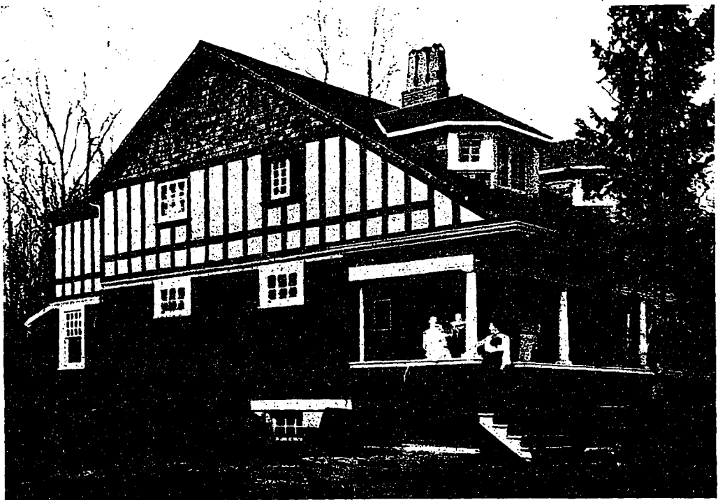
VIEW SHOWING SIMPLE AND EFFECTIVE TREATMENT OF END WALLS. TWO FAMILY DWELLING, BALMY BEACH, TORONTO. MR. CHAS. F. WAGNER, ARCHITECT.
