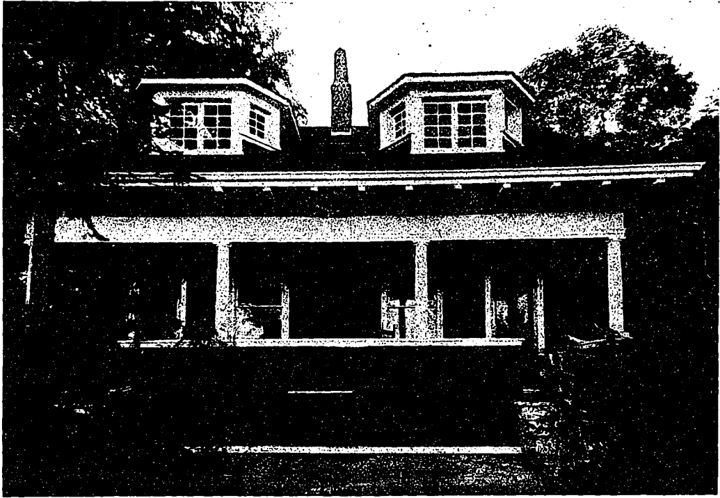
ATTRACTIVE TWO FAMILY DWELLING, BALMY BEACH, TORONTO. OWNED BY DR. J. W. ROWAN. MR. CHAS. F. WAGNER, ARCHITECT.
