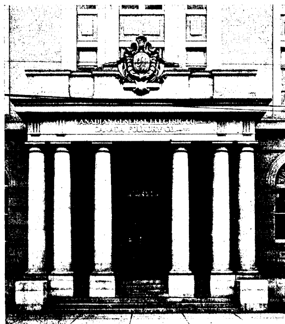
Main Entrance, Canadian General Electric Co.'s Building, Toronto. Darling & Pearson, Architects. FRED HOLMES & SONS, Contractors.
