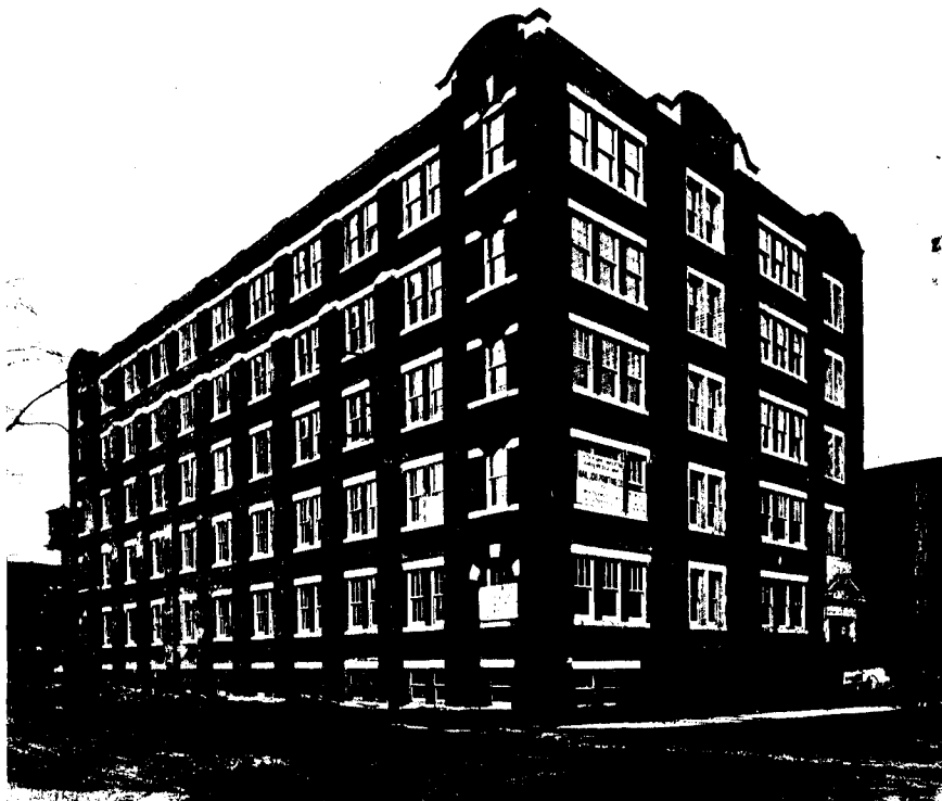
New Concrete Building for Mail Job Printing Co.
