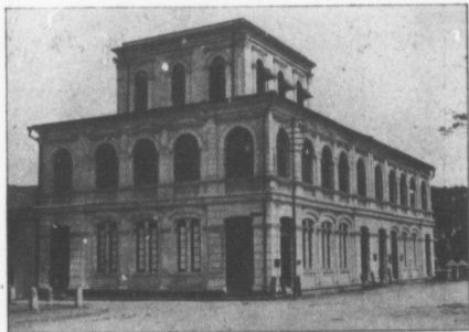
Office Building of Darley, Butler & Co. General Agents for Ceylon of the Sun Life Assurance Company of Canada.
