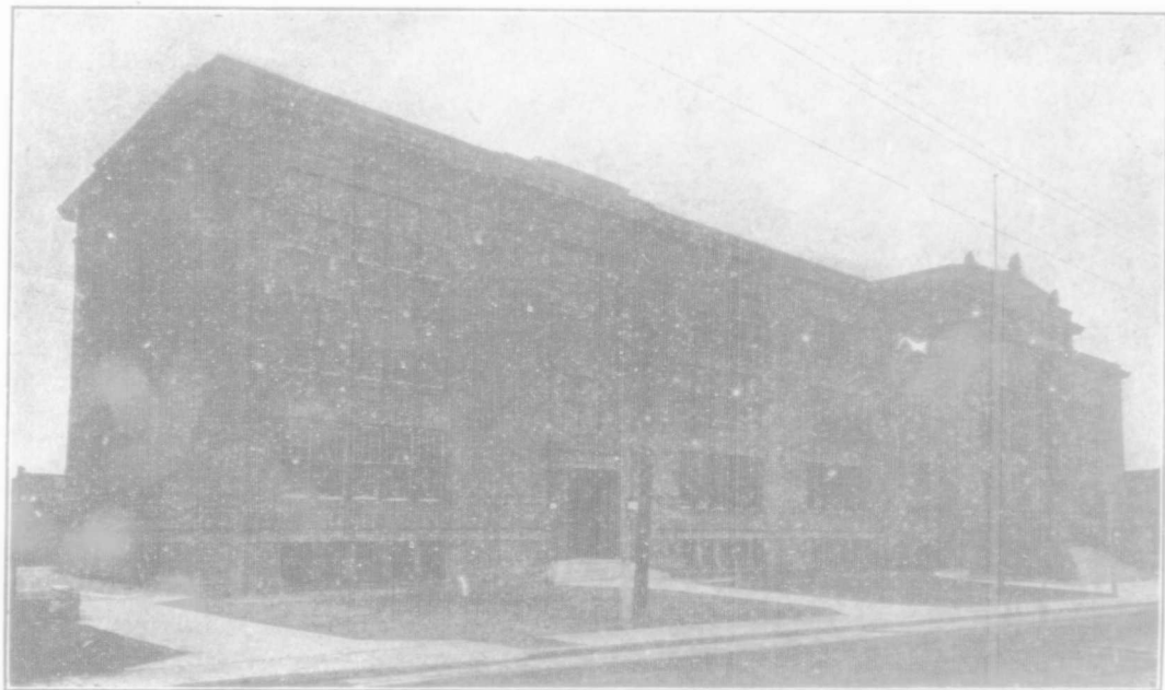
THE NEW PARK SCHOOL
