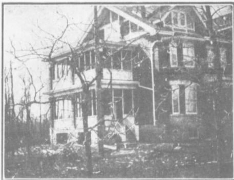
THIS SCREENED-IN VERANDAH IS A GOOD PLACE TO SLEEP
