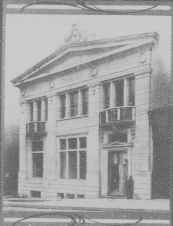
CANADA PERMANENT BUILDING Richards Street, constructed of Granite, supplied by KEAST & ALLEN, Stone Contractors , Works at False Creek
