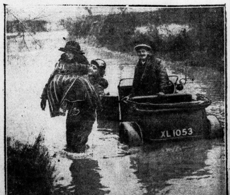
A passenger being rescued from a car caught in the flood in the Thames Valley, England.
