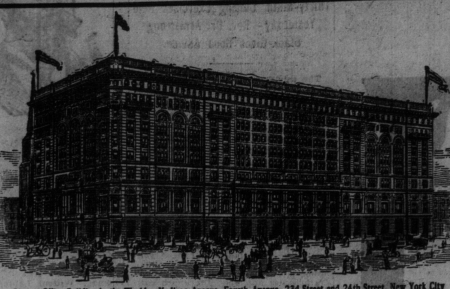
Largest Office Building in the World—Madison Avenue, Fourth Avenue, 23d Street and 24th Street, New York City
