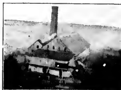
THE SUMNER CO.'S MILL AT BATHURST.
