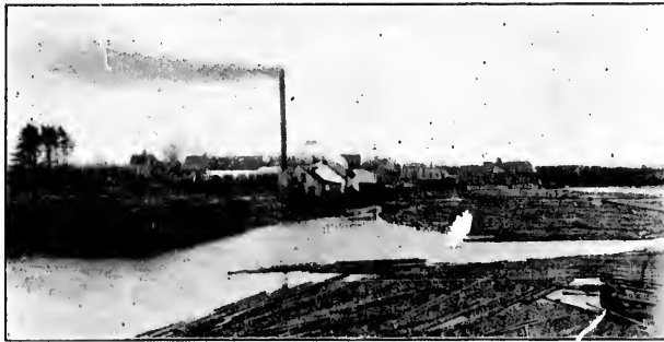
W. MASON & SONS' MILLS, BAYSWATER, OTTAWA.
