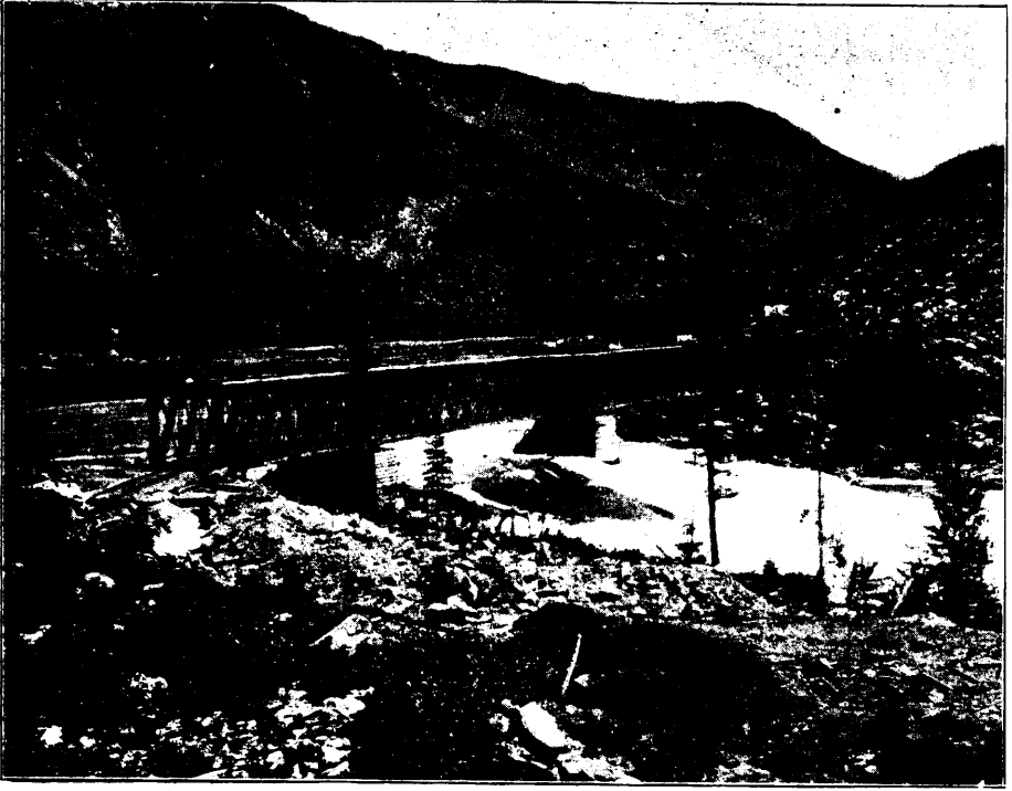
RAILWAY CROSSING OF THE KOOTENAY, NEAR NELSON.
