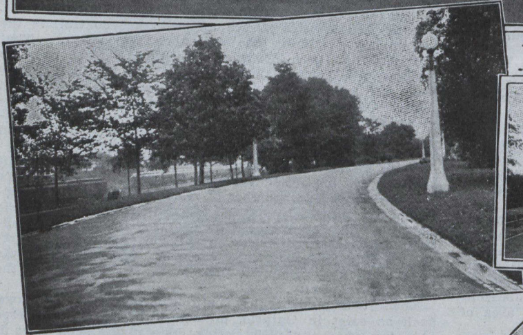
Rideau Canal Drive, Waterbound macadam road maintained with "Tarvia-B"
