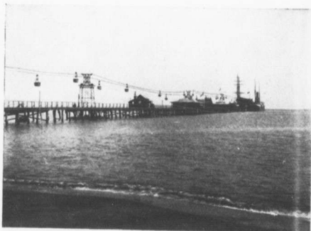
Loading Asphalt from Pitch Lake to Ocean Steamer—Trinidad.
