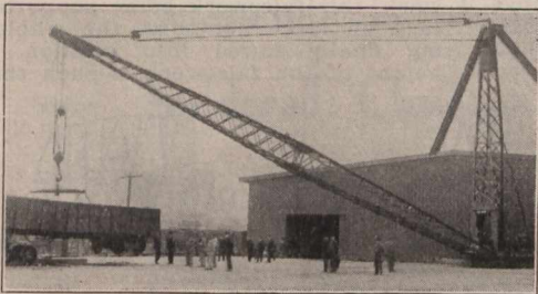
Oregon R.R. & Nav. Co. Albina, Ore., 35 ton "American" Steel Stiff Leg Derrick
