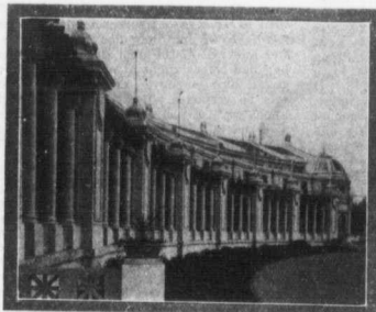
PERGOLA OF AGRICULTURAL BUILDING
