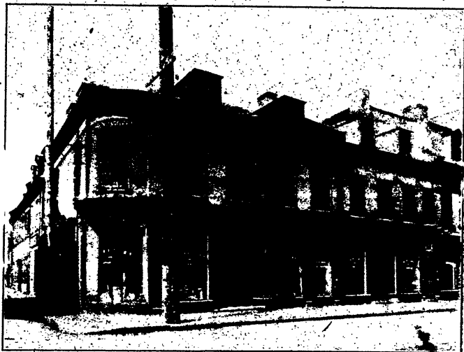
Heating, Plumbing & Electrical work
