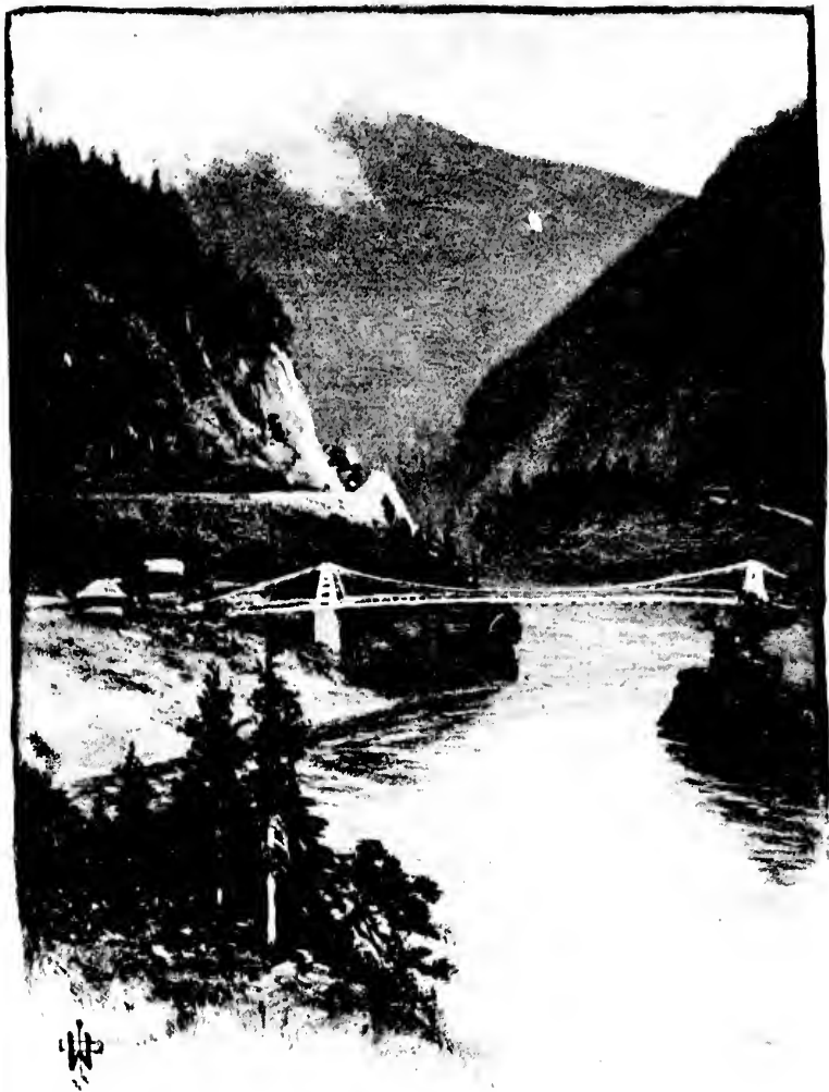
CARIBOU ROAD BRIDGE, FRASER.
