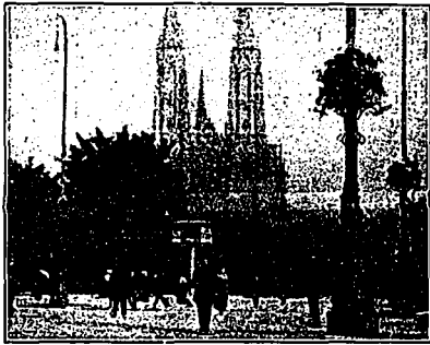
7.—Ornamental Tramway Poles, Vienna.
