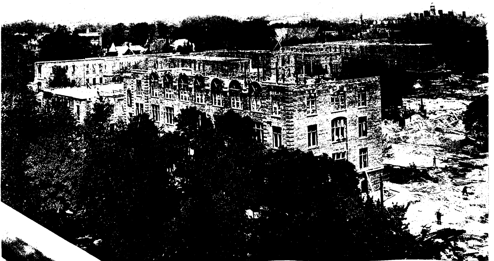
General view of the present state of the buildings under course of construction—Toronto General Hospital, taken from an elevated point of view on Spadina Ave., south of College St. Reference to the perspective shown on the opposite page will give an idea as to the location of the various buildings and how the group will appear when the work is completed. The walls with their panels, window arching, quoins, etc., all built in Don Valley J.A.P. Semi-Vitreous Brick, present a most charming effect. Darling and Pearson, Architects.
