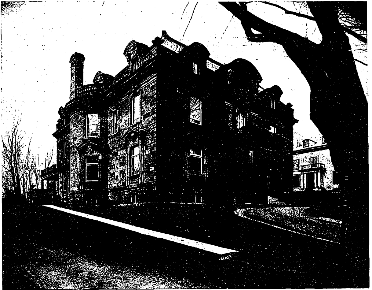
View from Main Approach, Montreal Residence.—Designed by Messrs. E. &amp; W. S. Maxwell.
