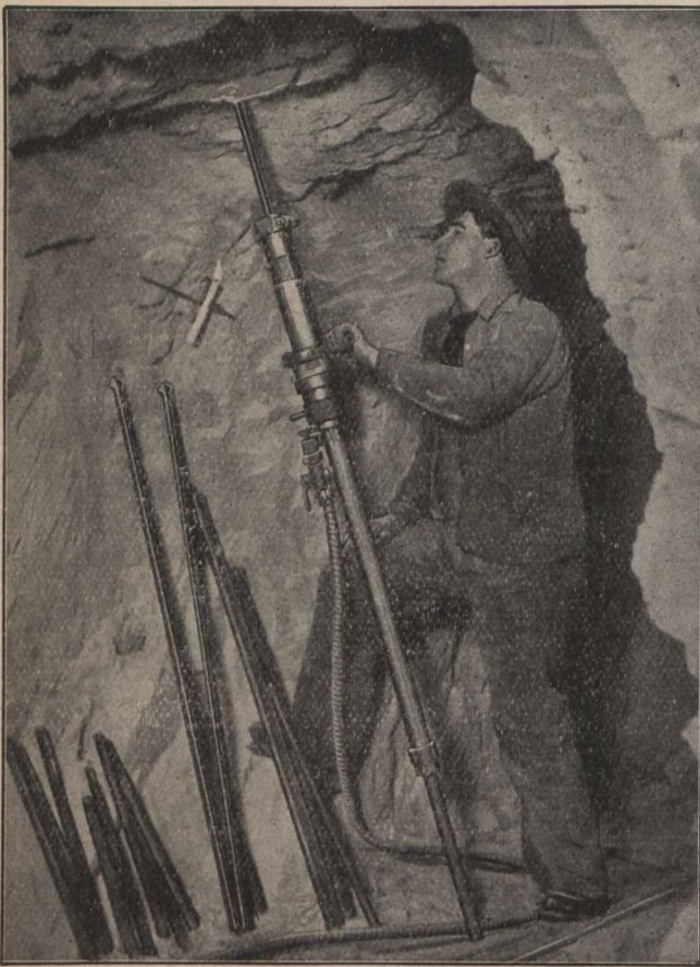
Sullivan "D-21" Hammer Drill in operation.
