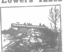
This picture of the Pedlar Perfect Culvert assembled and ready to lower into place, shows the immense strength and rigidity of these Culverts. Though forty feet long with a bearing of only a few feet at the centre it does not give one sixteenth of an inch. See how one-sixteenth of an inch. See how easily Pedlar Culvert can be lowered into place. No skill needed.
