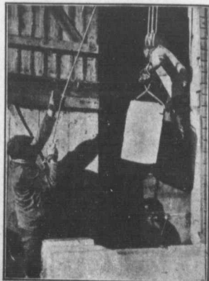
The Block and Tackle Lightens the Work of the Ice Harvester.
